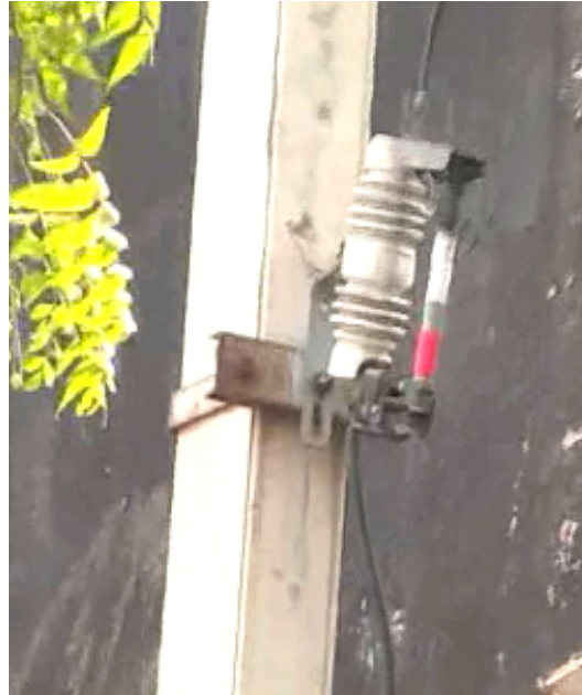
Lightning Arrester
